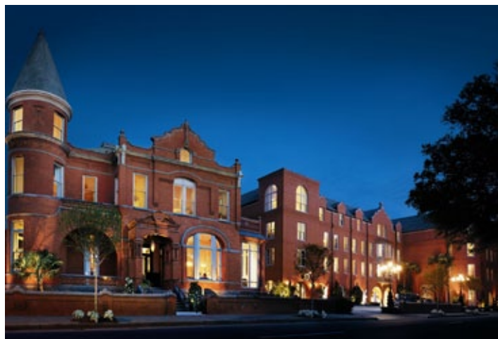
700 Drayton Street is also known as the Kayton-Grainger-Huger House, designed by architect Alfred Eichberg. The house is now part of the upscale hotel, the Mansion on Forsyth Park.
