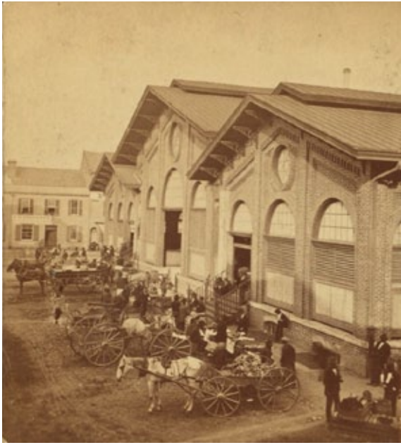
The original City Market building was demolished in 1954 to make way for a parking garage.
